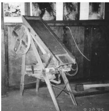
Dry wash placer machine used in central Nevada around 1910
